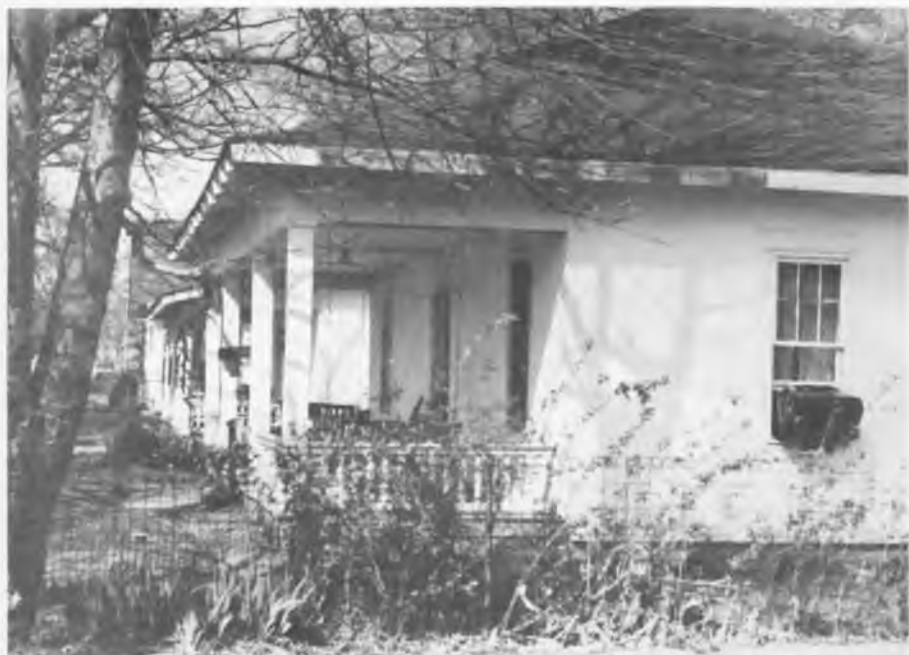
10. These mill-worker's rental houses on north Meridian street were probably built in the early 1920's by Lincoln Mills. While small and modest, they display the bungalow characteristics of wide, low eaves with exposed rafter-ends, wide front porch and rough-cast stuccoed walls. In its squarish hip-roofed form, these bungalows are actually closer to the original Bengali "bangala" than most of the more elaborate Swiss-influenced versions.
