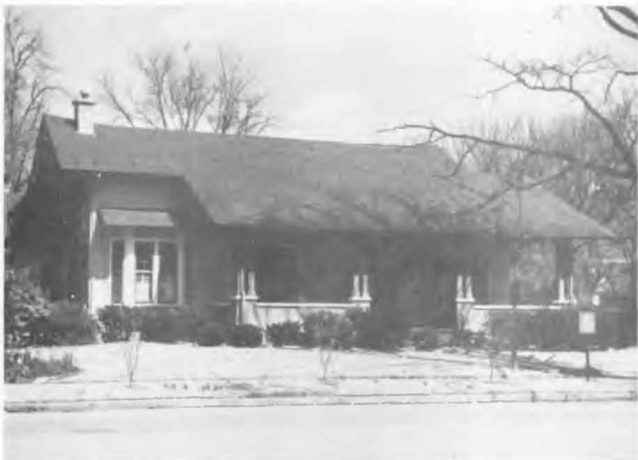
5. This fine early bungalow at 531 Franklin Street was designed in 1909 by the Huntsville architect Edgar Love. Notice the "kick" of the roof-ridge ends - a refinement found in at least one other Huntsville bungalow. The zig-zag roof and bay window give this bungalow an informal and welcoming air.
