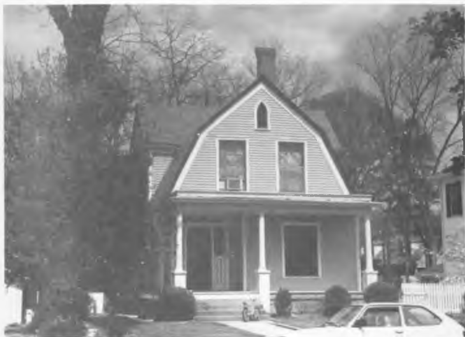
2. This 1901 house at 603 Franklin Street by the architect Herbert Cowell has a Dutch-Colonial Revival gambrel roof combined with late-Victorian massing (vertical, narrow, irregular). A small "Gothic" vent is in the gable. The windows are quite wide and squarish in proportion, unlike those in the Victorian styles. A balustrade once ran along its porch roof, as evidenced by the base for it, and there may have been a balustrade also at the porch floor level that ran between the masonry piers which support the porch columns.
