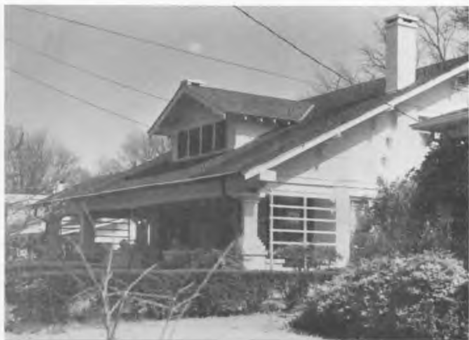
9. This 418 Locust Avenue 1922 bungalow exhibits the Swiss influence (long, low swooping roof, large dormer, stucco, false half-timber) but not in a literal manner.(3) Notice the "missing" porch columns - a deliberate design feature. It would be an error to "replace" them. This house was built by Fisk & Hopper, contractors. Its design probably came from a "bungalow book" of stock plans.
