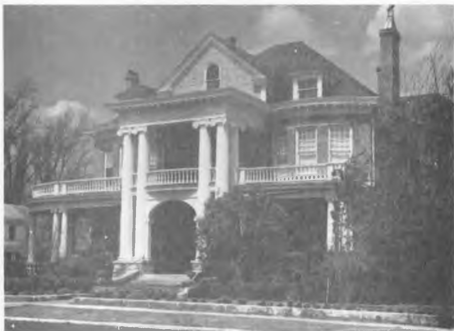
3. This finely-detailed, well-constructed ca. 1902 house at 501 Franklin Street was designed by the architect Herbert Cowell. It is an amalgam of mostly classical elements such as Ionic fluted columns, Adamesque frieze, modillioned cornice, balustrades etc., with some holdover influence of the Victorian period as seen in the broken flowing massing and the chimneys with vertical inset ribs - a Queen Anne device, as is the pebble-finish tympanum and use of stained glass. This house is a very free, unacademic expression of predominantly Colonial Revival elements which might best be called "Free Classic" in style, a recognized term of the period.
