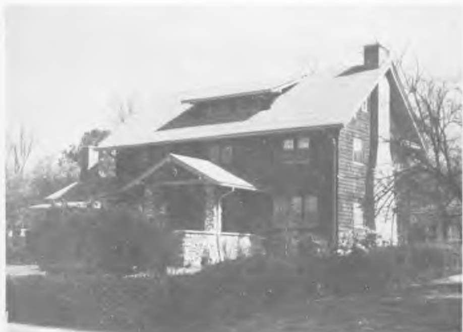
6. This 1914 house at 612 East Holmes Avenue could be termed a "Swiss style bungalow". It bears a strong family resemblance to many 17th and 18th century Swiss rural houses, with its use of fieldstone, natural wood shingles, and steep gabled roof. The wide, low shed-roofed dormer is also found on old Swiss houses.(3) These Swiss forms, including the use of rough-cast stucco and false half-timber, are found on many bungalows and it would be fair to say that old Swiss houses were a major influence on the bungalow style.
