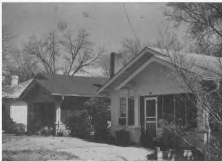
This pair of small identical bungalows at 430 & 432 Locust Ave. were built in 1923. They were probably built from stock plans on speculation, as many houses were in this boom period. The front porches were likely enclosed later, for screened front porches were not common in this period. The builder of these houses is unknown.
