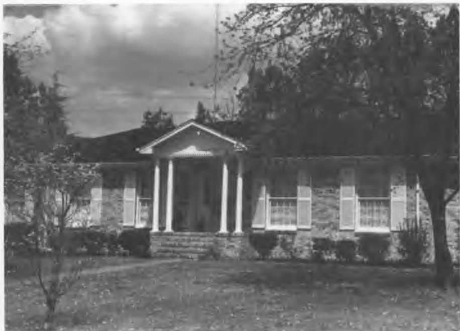
14. This 1960's house on Lucerne Drive is one of Huntsville's many latter 20th century "Ranch-Colonial" examples. This one unwittingly relates very closely to the designs of the 16th century architect Andrea Palladio (see text) and thus is a good candidate for the term "Ranch-Palladian". The design may be from a stock plan, or from a "house-plan service" (local drafting companies that work up plans for speculative builders, usually as modifications and variations on the builders' favorite plans). This neighborhood has several houses of nearly-identical plans, but with exterior variations and "reverses".
