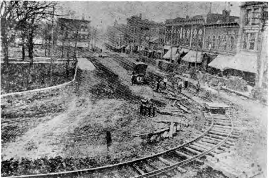
East Side Square, laying of street car track, 1902.
