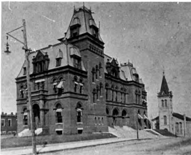
Federal (Postoffice) building, Huntsville, completed in 1890, at the intersection of Eustis, Greene and Randolph Streets. It was razed in 1954.
