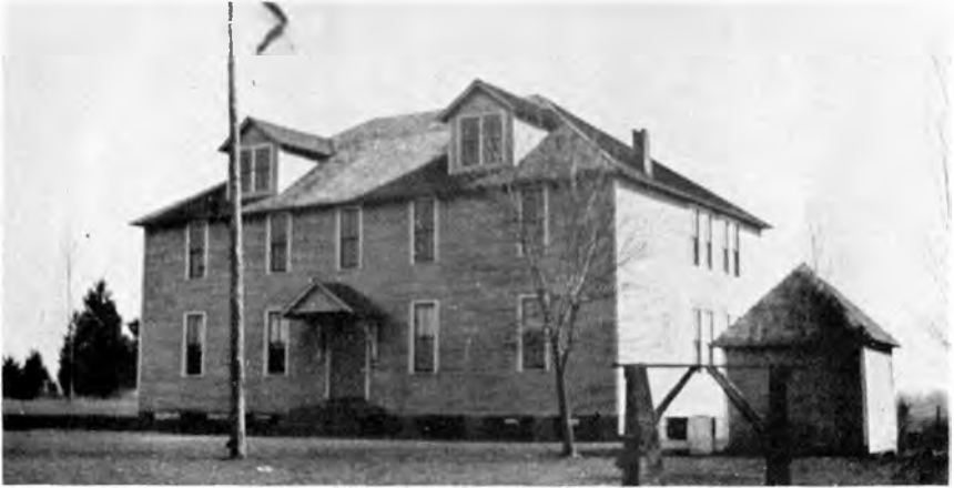
Meridianville High School, 1924, on site of former school which burned
