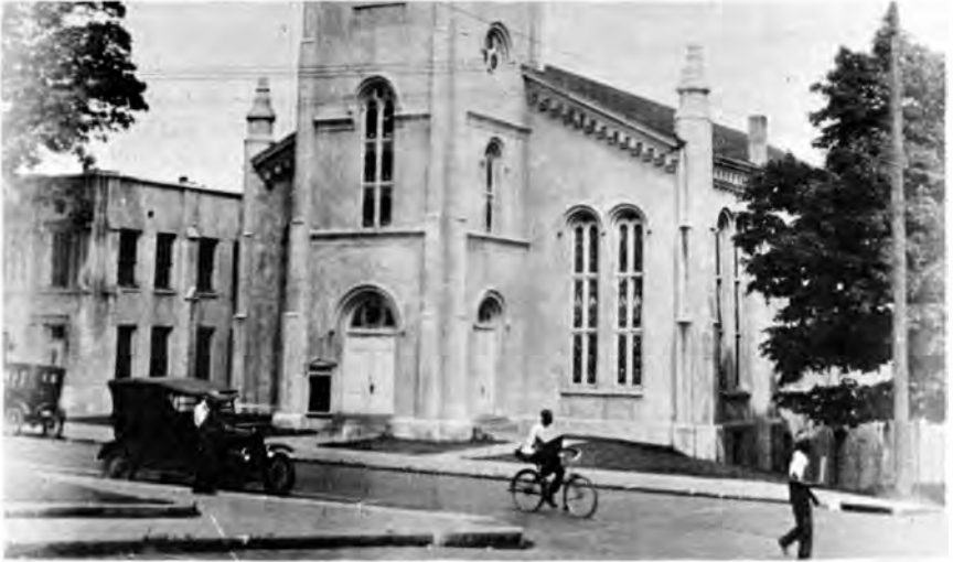
First United Methodist Church. First building, built on present site in 1833, burned by Union troops in 1864. Present building cornerstone laid 1867.
