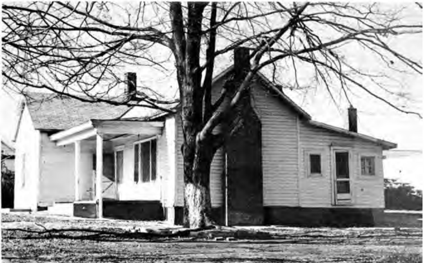
1972 view of building on Pearl Street, that served as one of the first suburban schools in Madison County.
