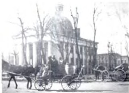
Madison County Courthouse
