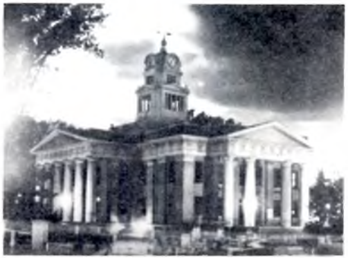
Madison County Courthouse 1914-1964
