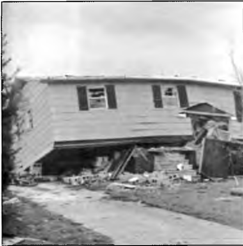
One of the homes destroyed by a tornado
