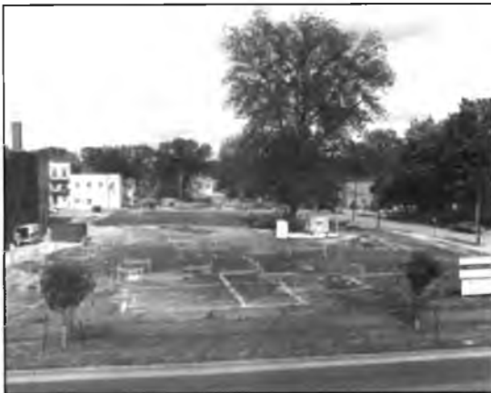
Constitution Hall Park being laid out
