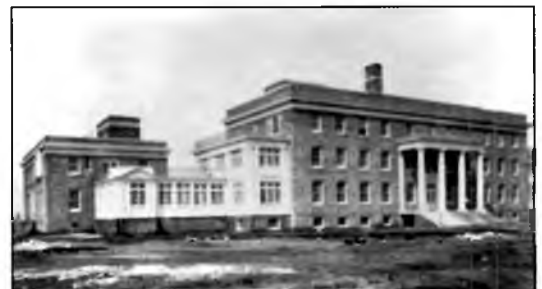
Huntsville Hospital upon completion
