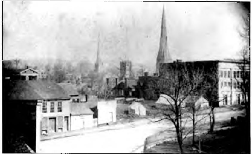
East Side of the Square
