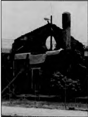
Freight Depot Destroyed by Fire
