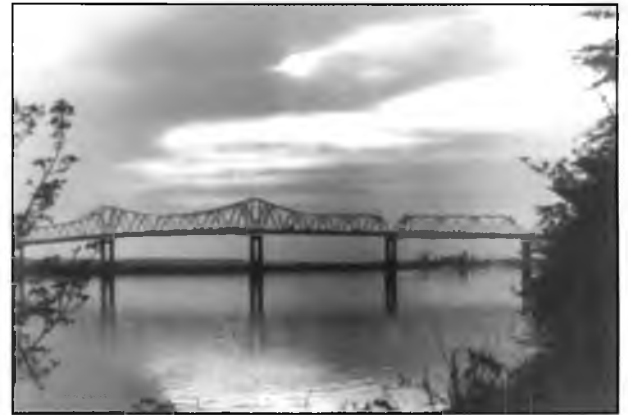
Clement C. Clay Bridge
