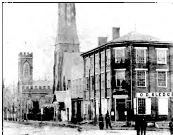
Kaufman Building is next to the Episcopal Church
