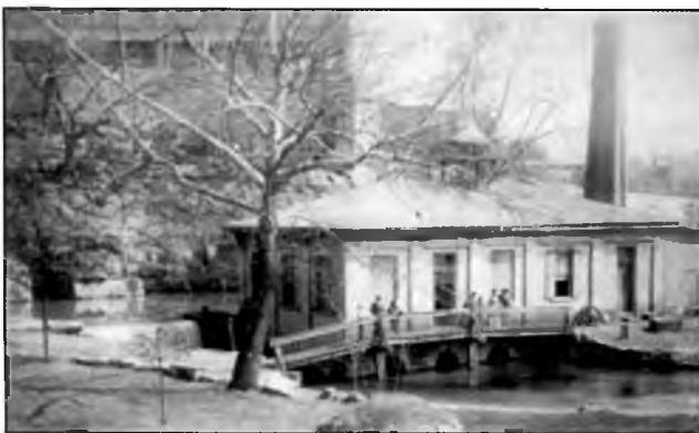
Big Spring Water Turbine
