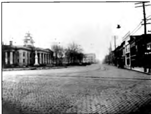
Brick Paving Around the Square
