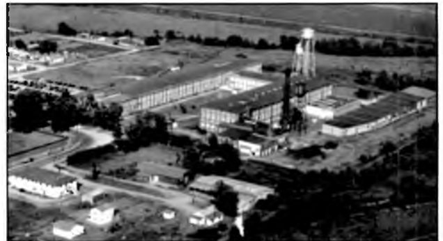
Lowe Manufacturing Building
