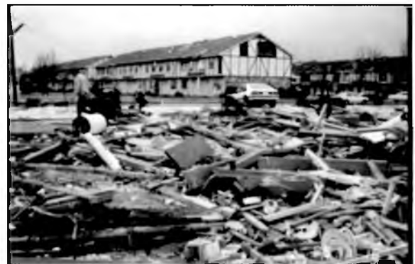
Destruction on Airport Road
