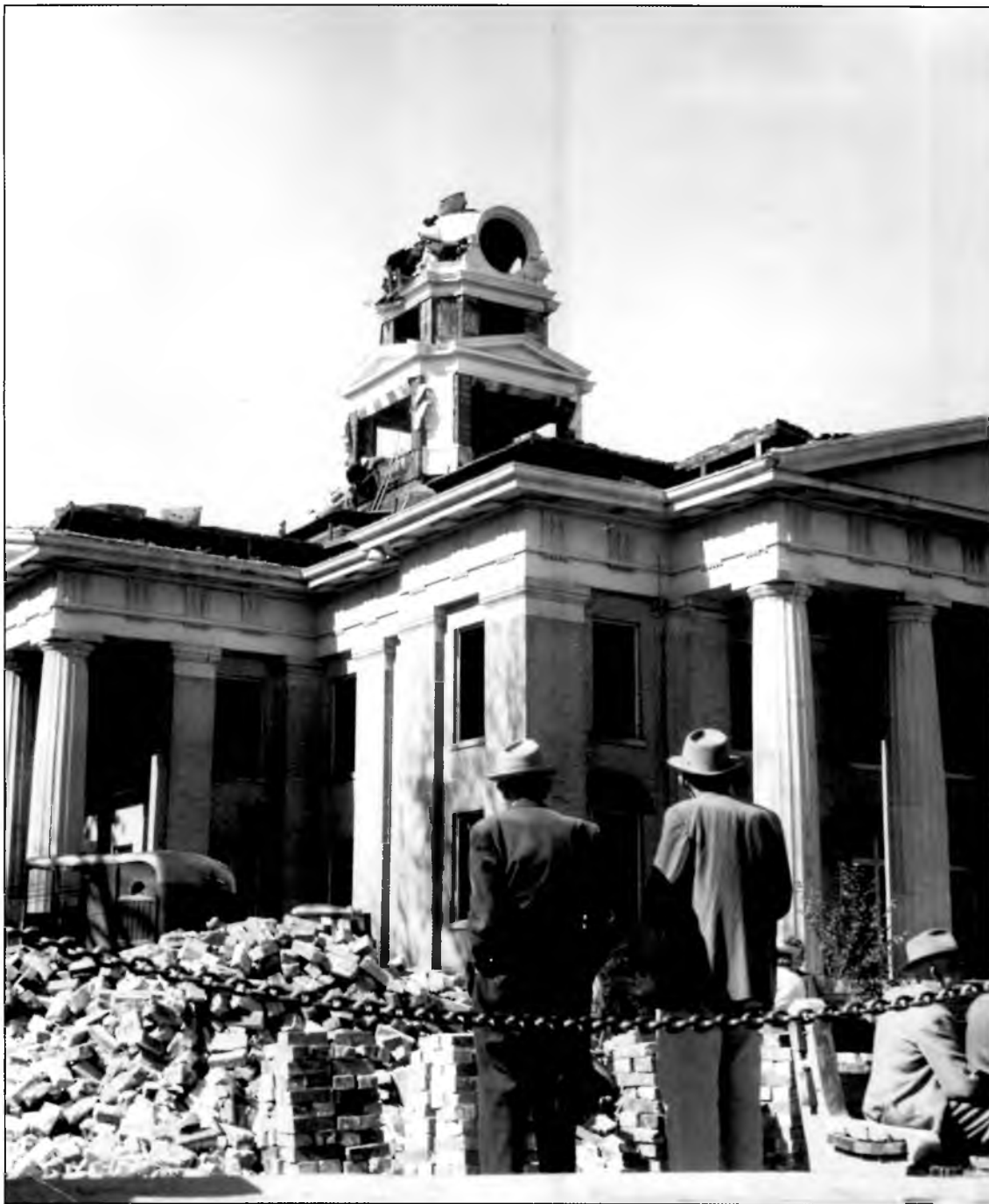
Old timers watch as the courthouse is being demolished in the fall of 1964. The weathervane atop the dome was moved to what is now Regions Bank. Some of the 20 Doric columns mark the entrance to Huntsville Botanical Gardens.
