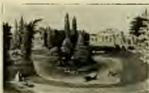
"Gaineswood" estate of Gen. Nathan B. Whitfield, near Demopolis
