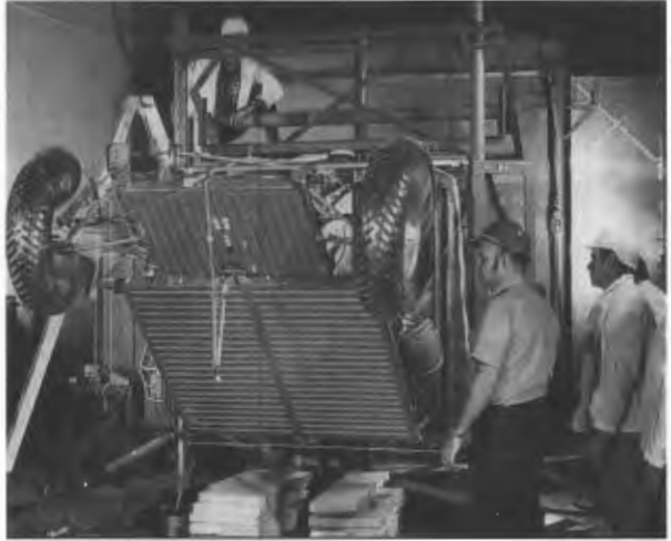
Deployment testing of lunar roving vehicle in March 1971.
