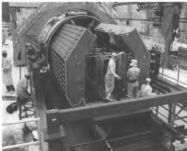
Spacelab 3 rack/floor installation at KSC in May 1984.
