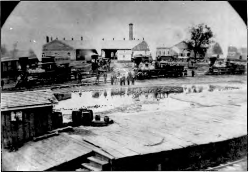
Huntsville Roundhouse - Troops and supplies were delivered and trains rerouted here. Remains of spring flooding can be seen. HMCPL.
