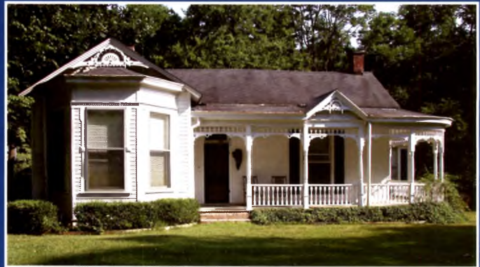
310 Martin Street, Lanier House
