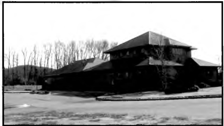
Grace Presbyterian Church on Wall-Triana Highway, photo made 2002
