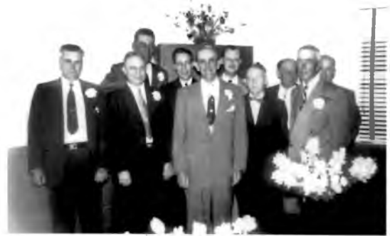
1955 dedication of third City Hall, now Main Street Cafe. (L-R) Police Chief A. V. Kay, Commissioner Caudis H. Tribble, Builder Redus H. Riddle, City Attorney M. H. “Pete” Lanier, Mayor Howard Dublin, Baptist Preacher R. W. Thompson, Methodist Preacher Guy E. Wallace, Water Department Supervisor W. C. “Bill” Gillespie, Commissioner Charles F. Apperson Sr., City Clerk Robert E. “Pud” True.
