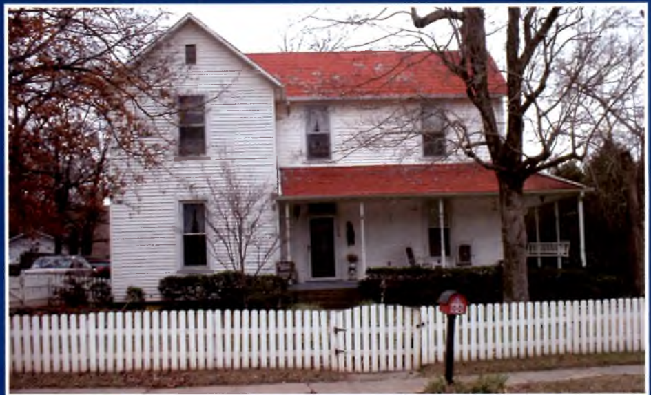
110 Church Street, Keebler House
