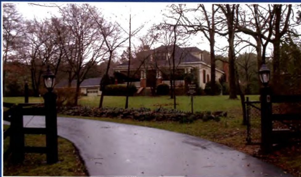
320 Martin Street, Bashore House
