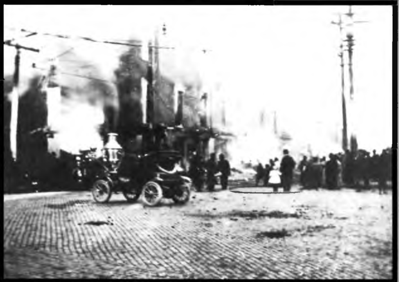
On the northwest corner of the Square, the Huntsville Hotel fire rages, November 11, 1910. Credit: George O'Reilly
