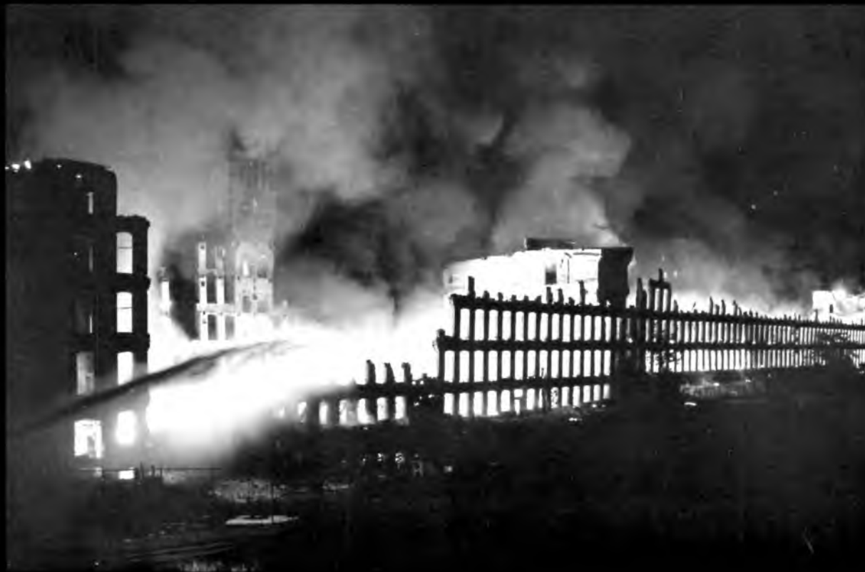
Early morning fire destroys the old Dallas Mill Building, July 24, 1991. Credit: Eric Schultz/The Huntsville Times
