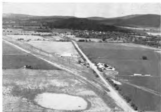
Intersection of Memorial Parkway and U. S. Highway 38 near Lily Flagg Community during early period of Parkway construction.
