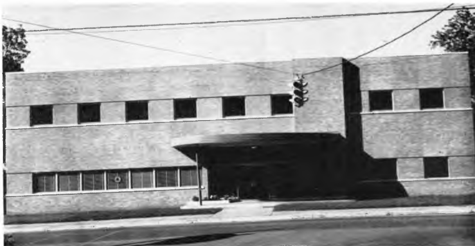
Above is telephone building which houses Southern Bell offices and equipment needed to operate Huntsville's new dial system installed in 1954 at a cost of $2 million.
