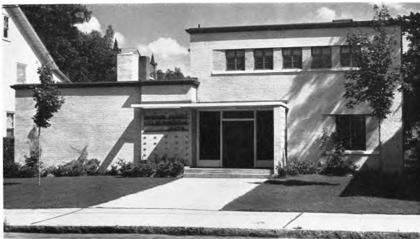
Madison County-City of Huntsville Health Center.
