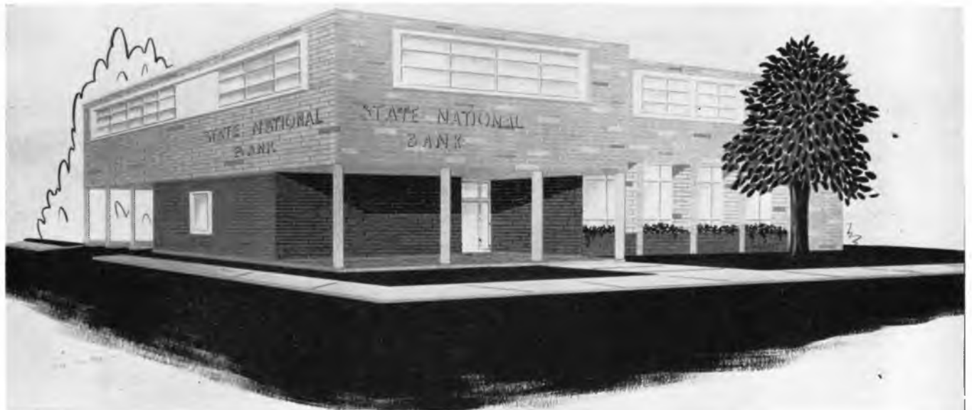
New State National Bank building under construction
