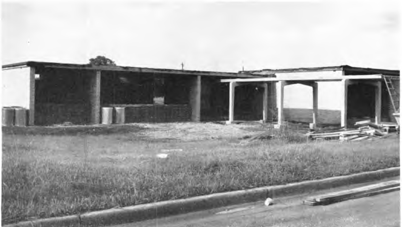
Crippled Children's Center under construction.
