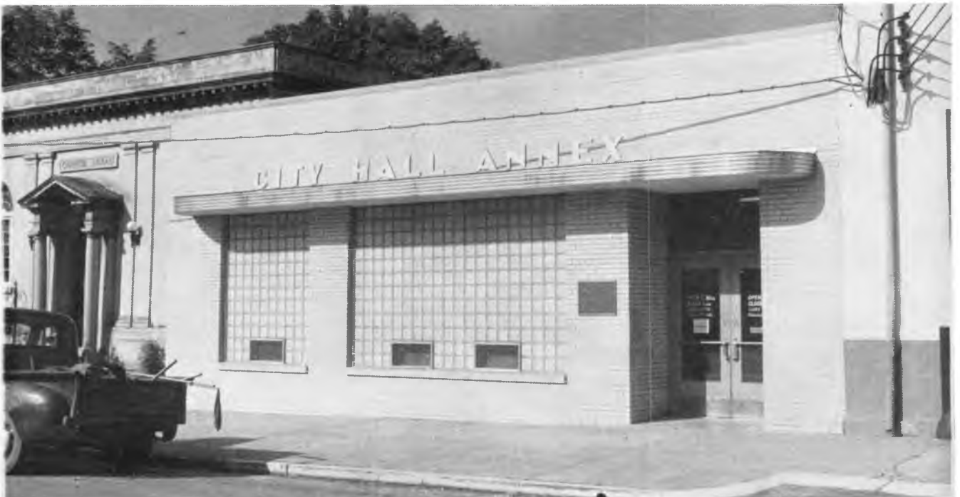
City Hall Annex
