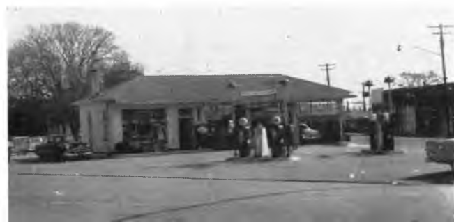
Ashby Service Station
