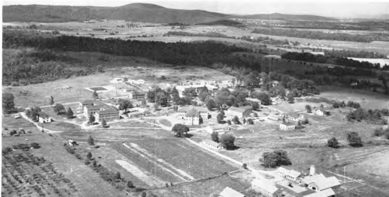
Aerial view of Oakwood College
