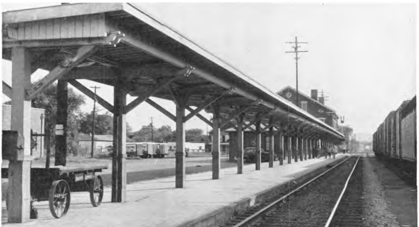
Southern Railroad Depot
