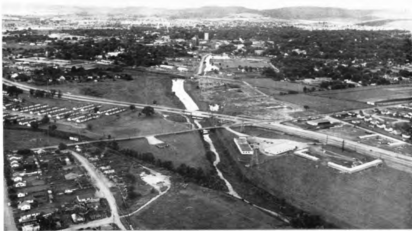
View of multi-million dollar Parkway now under construction
