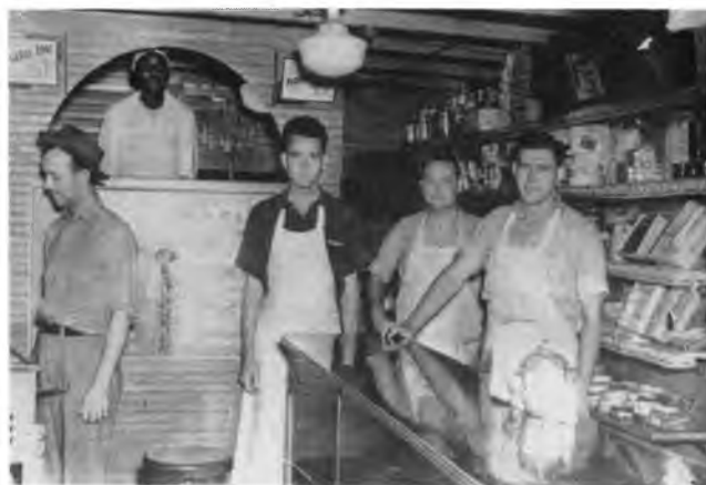
Interior view Clark Steadman's
