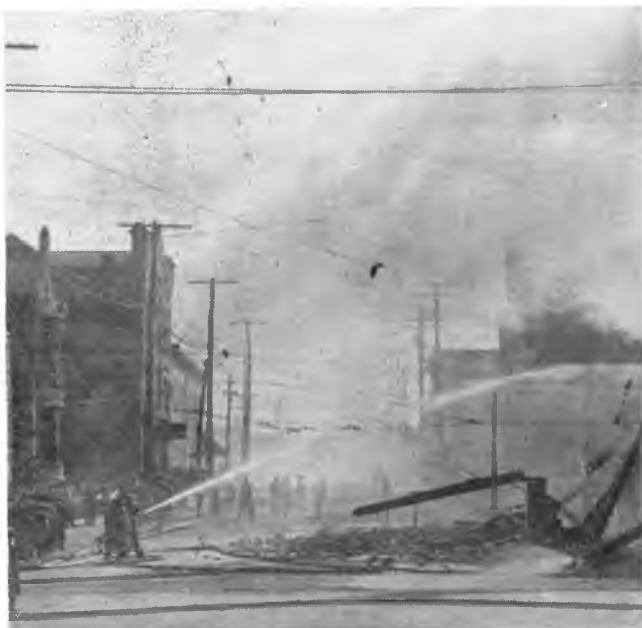
Opera House fire (Courtesy picture)
