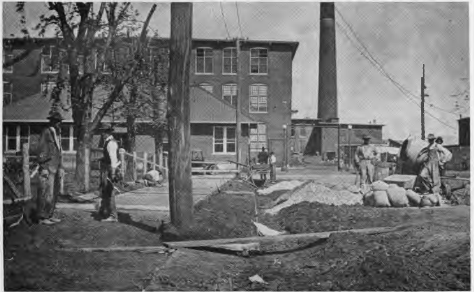
This view of sidewalk construction was taken on April 22, 1920. Howard Jones was foreman of this construction work. Sidewalks and curbs were laid all over the village by the company. It was five years after this that the county paved Triana Pike.
