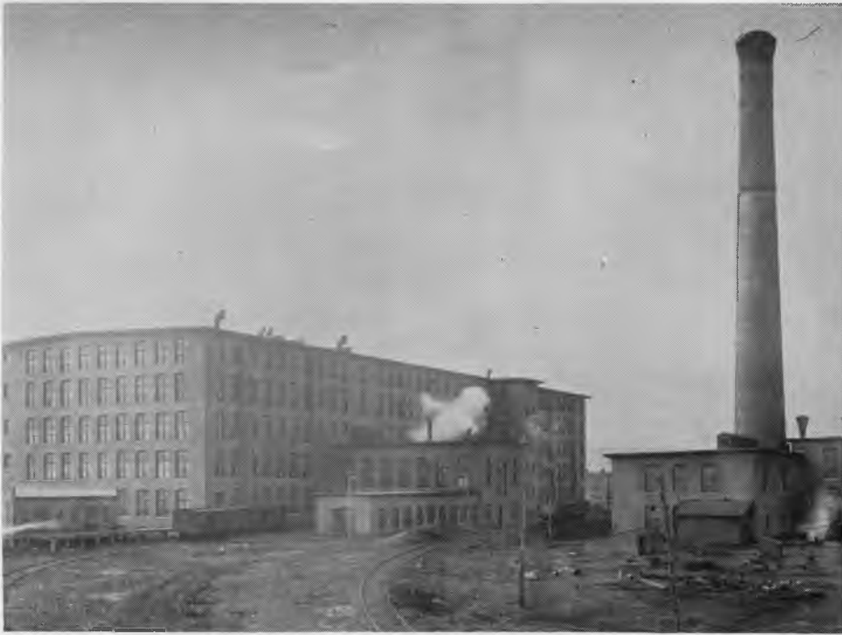
This photograph was taken about 1904 or 1905, shortly after the plant began operating. At that time the clothroom was separate from the mill. Cotton was stored on the first floor of the mill in these early days. A coal car can be seen on the trestle that ran between the mills.
