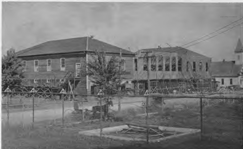
This photograph, made on September 18, 1920, shows the beginning of the brick store buildings. The frame building already on the corner was left standing and the architecture of the new building fitted to it.
