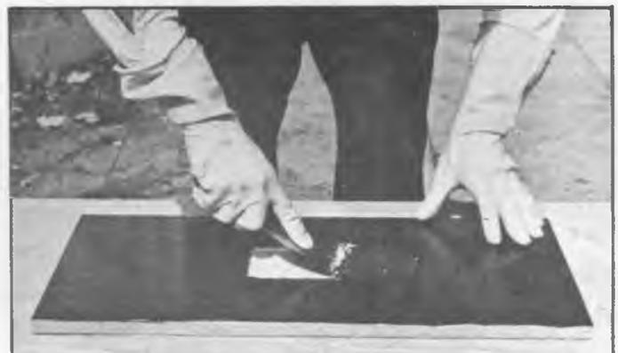
Remover is allowed to soak in until a wide-bladed putty knife can scrape off all paint layers in a continuous ribbon. If necessary, more remover is applied until scraper can cut through to clean wood.
