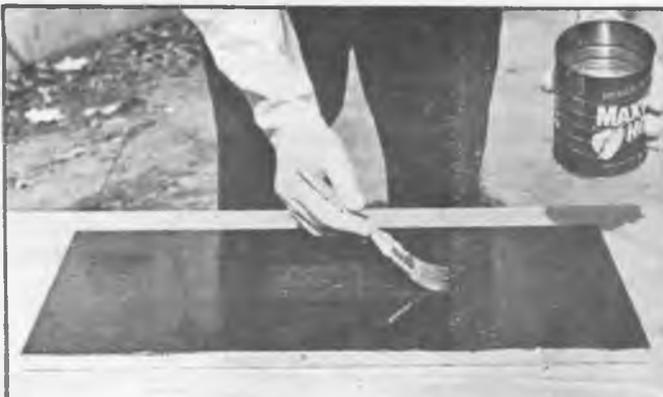
Remover is laid on thickly, using as few brush strokes as possible. Rubber gloves protect hands from burns. If remover starts to dry out before all paint is loosened, the area is re-soaked.
