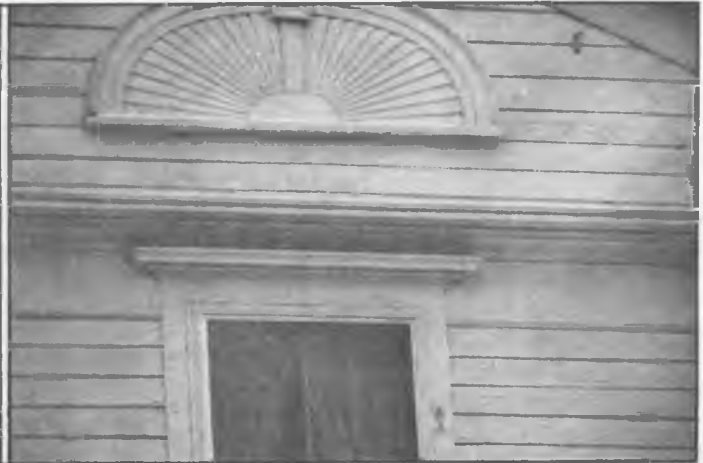
dow and created the cap on the window cornice to match the original woodwork (shown on the window at the right).
