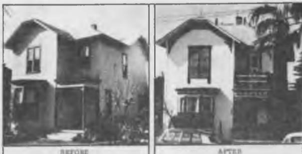
Exterior restoration included ripping off the asbestos shingles and repainting, installing finials at roof peaks, creating a widow's walk atop the house, re-creating much gingerbread trim, and replacing the door and railing for the small second-floor porch over the front door.
