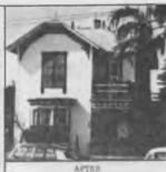
Exterior restoration included ripping off the asbestos shingles and repainting, installing finials at roof peaks, creating a widow's walk atop the house, re-creating much gingerbread trim, and replacing the door and railing for the small second-floor porch over the front door.
