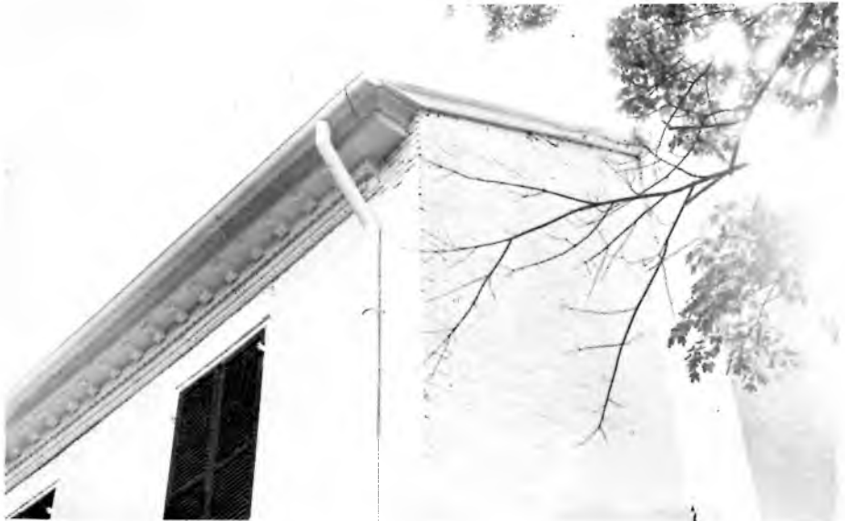
Cornice and gable wall of WEEDEN House.
