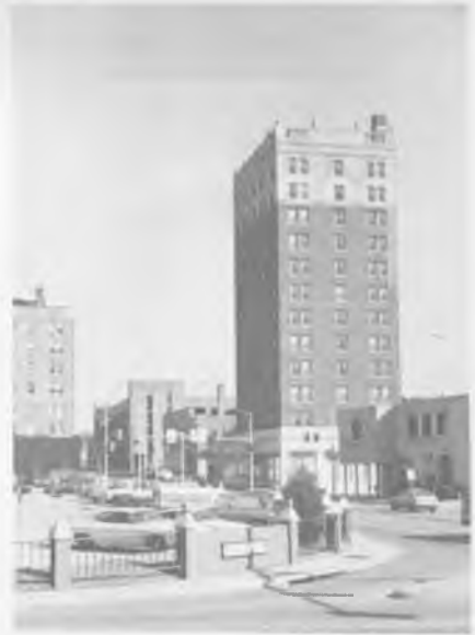
Russel Erskine Building
