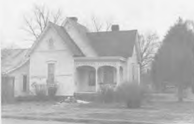
Bierne Ave. A Victorian "Carpenter Gothic" being restored.
