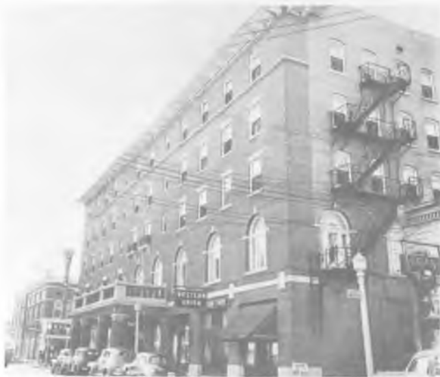
Hotel Twickenham, Clinton Avenue view. Built 1914, demolished 1975.
