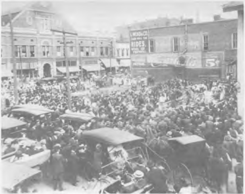
Groundbreaking for the Hotel Twickenham, April 23, 1914.
