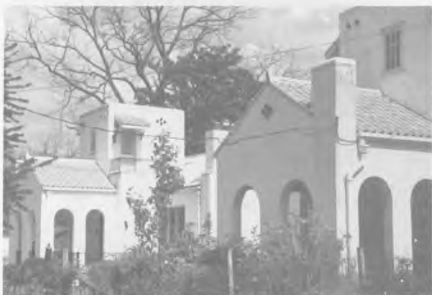
This pair of nearly-identical stuccoed houses at 136 and 138 Walker Avenue represent the Spanish Colonial Revival style, rare in Huntsville but very common in some other cities. They were built in 1929 by Harold Riggins. The ceramic pan-tile roofs are probably the 56-year-old originals. These small houses are unusually good examples of their style.
