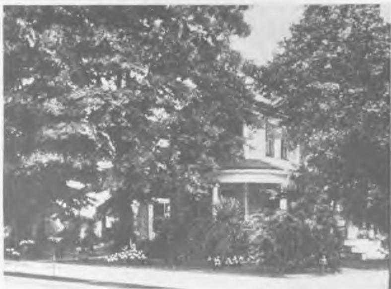
516 E. Holmes Avenue. The old Suggs Home. This house burned in 1976.
