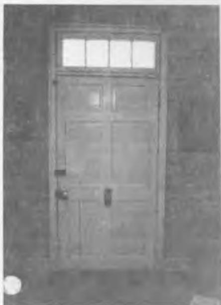
**LEFT:** The front doorway has a Federal six-panel door with the old rimlock still in place, plus a transom above. The door panels are raised on the interior side and flat on the exterior. Baseboards are of the narrow Federal style, although quarter-round and toe mouldings have been added at top and bottom.
