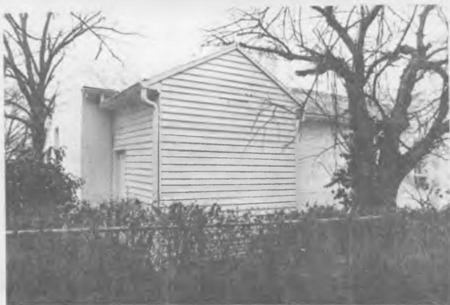
This frame addition at the northeast end of the brick house was apparently built during the Federal era. Note the tapered rake fascia (boards forming an angle at the gable), the boxed eaves, and the uneven clapboard.
