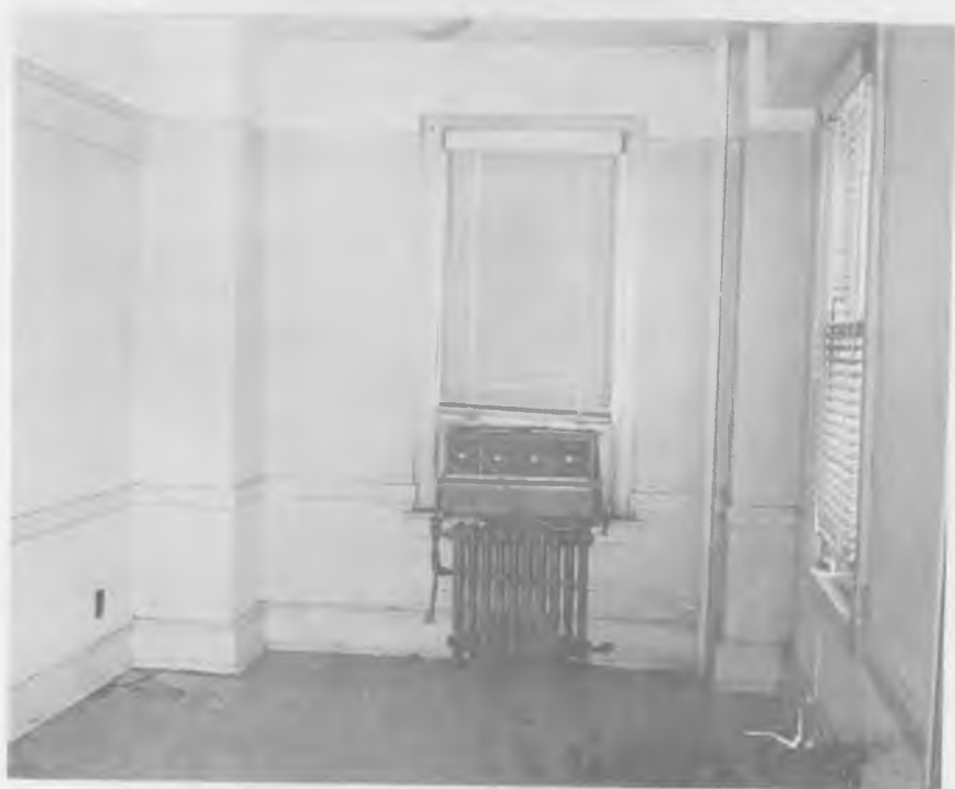
Notice the exposed plumbing for the radiator and how the concrete piers jut into the room.
