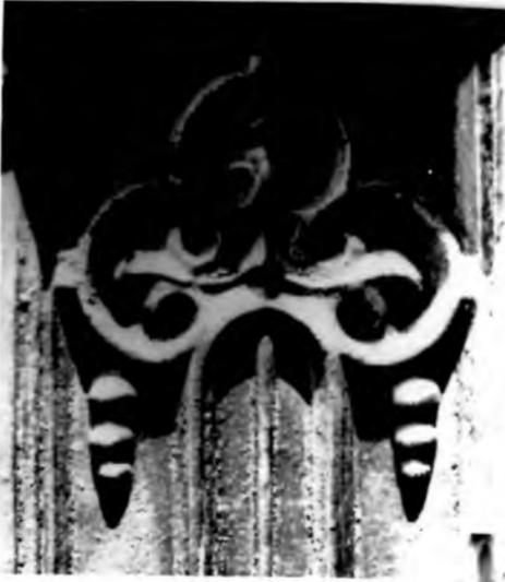
(4) The Church of the Nativity, 1859. Detail of ornament cast into the Gothic-Revival gatepost. This gatepost is an example of mid-19th century industrialization; an identical design can be found at a Mobile cemetery. Cast-iron building components in 1859 could be picked out of catalogues just as most parts for buildings are today.
