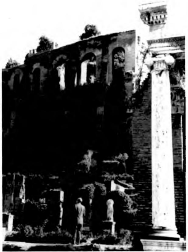
The best "art in architecture" is that which is inseparably integrated into the building elements rather than merely applied like an after-thought. A Greek ionic column is a structural member, yet it is much more. It is a work of high art, involving a sophisticated yet simple use of geometry in plotting the gentle swell of the column shaft, the spiral curve of the vaults and the elliptical cross-
