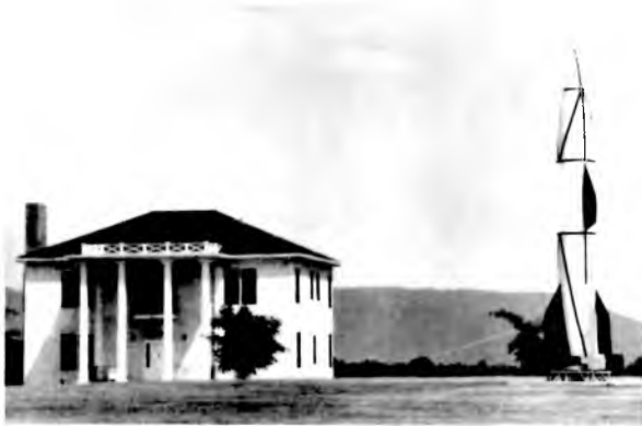
A Hermes missile is displayed in front of the house after its move to Redstone Road. This photo was made before the application of brick.
