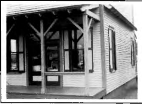
Window and door frames — at the Railroad Depot.
