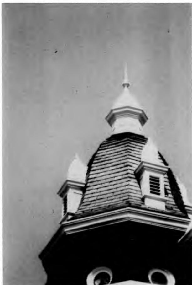
**Photo 2:** N.W. main tower with hand-worked sheet-copper finials replicated in 1994 to match the deteriorated 1899 galvanized-roof finials. The roof is gray slate.
