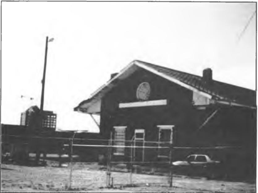
Let's just take a look at that building. It's falling apart, isn't it? The roof is a disaster, and most probably leaks. Bricks are falling out from around the foundation. Pigeons have nests throughout. Paint is flaking off all over. Wood is rotting everywhere. It certainly appears to be in need of a major overhaul. One might question whether it should be saved at all.
