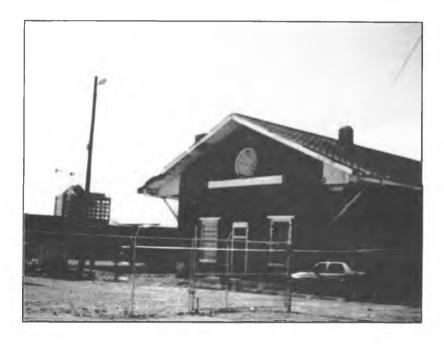
Let's just take a look at that building. It's falling apart, isn't it? The roof is a disaster, and most probably leaks. Bricks are falling out from around the foundation. Pigeons have nests throughout. Paint is flaking off all over. Wood is rotting everywhere. It certainly appears to be in need of a major overhaul. One might question whether it should be saved at all.
