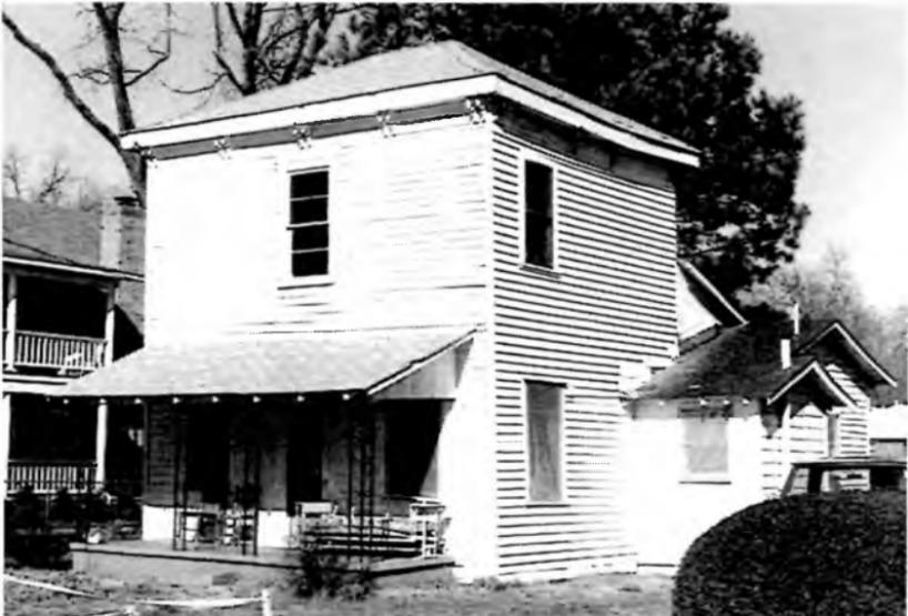
*February, 1991 photograph before restoration. Chimney is gone, original tall sashes replaced by short “ranch house” sashes, original veranda replaced by a makeshift shed, site filled-in about 12 to 18 inches deep, giving the house a stumpy proportion. Roof cornice-mould gone.*
