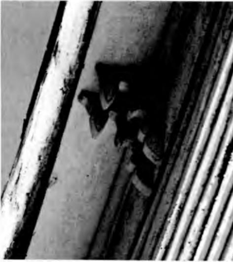
*LEFT: 1993 photograph of the unrestored roof cornice. The 1881 brackets, frieze, bed-mould and fascia remain, with only the top cornice-mould missing.*
