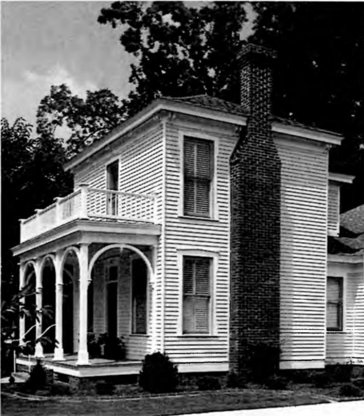
*1996 restored view. All is based on site evidences except the exact trim details of the veranda, for which no details remained. The 1996 addition is behind the house to the right, and the upstairs bath addition is tucked down into the attic of the first floor addition, barely visible at the upper right behind the 1881 second floor room.*
