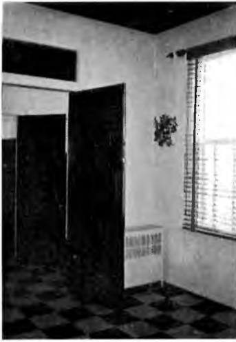
38. Looking south from the breezeway room to the 1924 butler's pantry.
