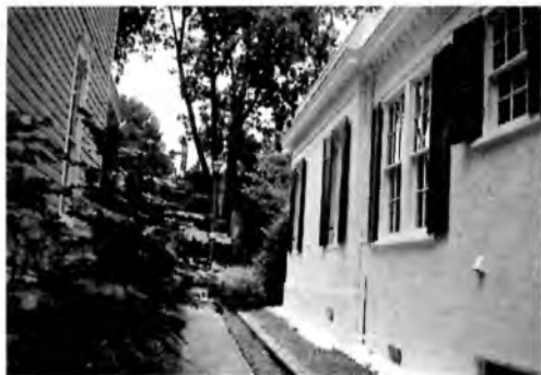
7a. After renovation, the A/C unit removed.
