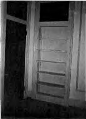
31. Southeast corner of the east room of the 1818 main body and detail of the 1924 radiator.
