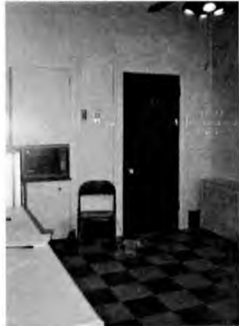
41. Detail of the 1924 decor of the 1883 kitchen wing.
