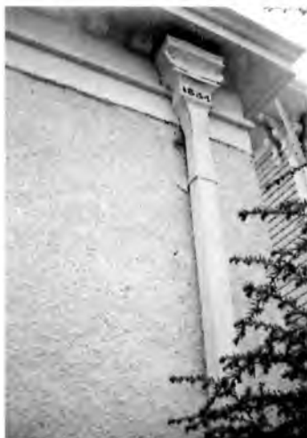
9. Front porch detail, Doric style column.
