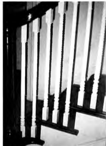
44. Detail of the balustrades.
