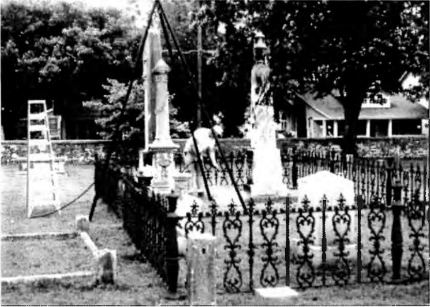
*Marker, Dr. Thomas Fearn plot, Maple Hill Cemetery, during restoration. Skip Stinson, masonry contractor by profession, artisan by interest, uses his self-designed tripod with chain hoist for dismantling, repairing and reassembling monuments.*
