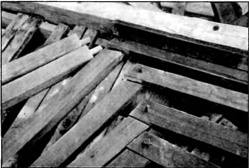
Fig. 4 Roof rafters, disassembled, Hollingsworth-Allen House, June 1995.
