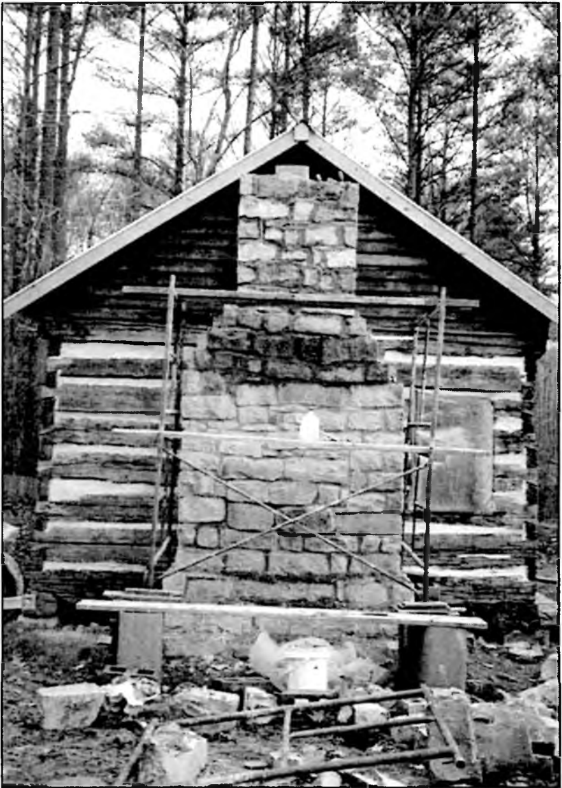
Fig. 8 Hollingsworth-Allen House, chimney rebuilding, December 1995.
