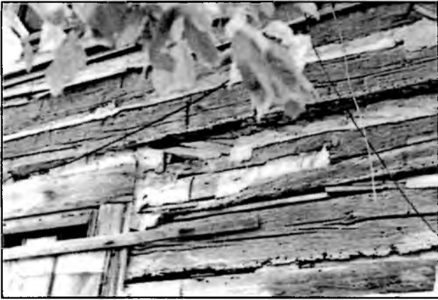
Fig. 11 Chinking detail, yeoman' house, Paint Rock Road, Madison County. Courtesy Debra Miller.
