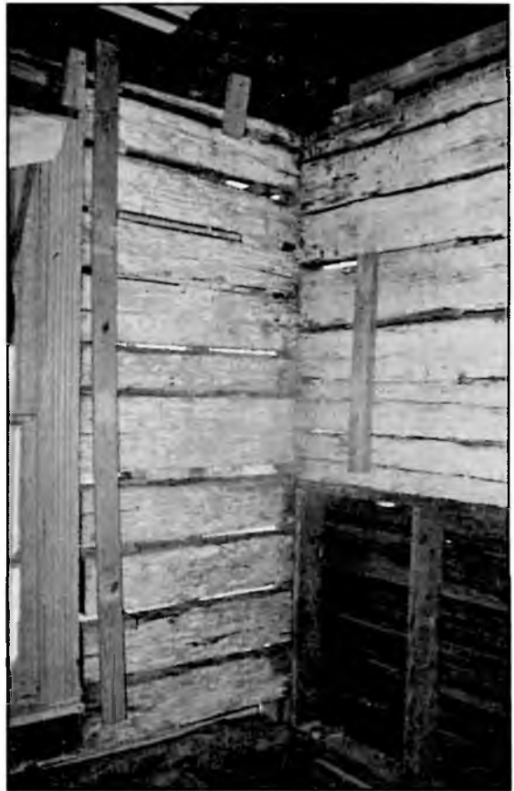
Fig. 6 Cabaniss-Ezell House, closeup of corner, repair in progress, late 1980s. Courtesy Gene Ezell.
