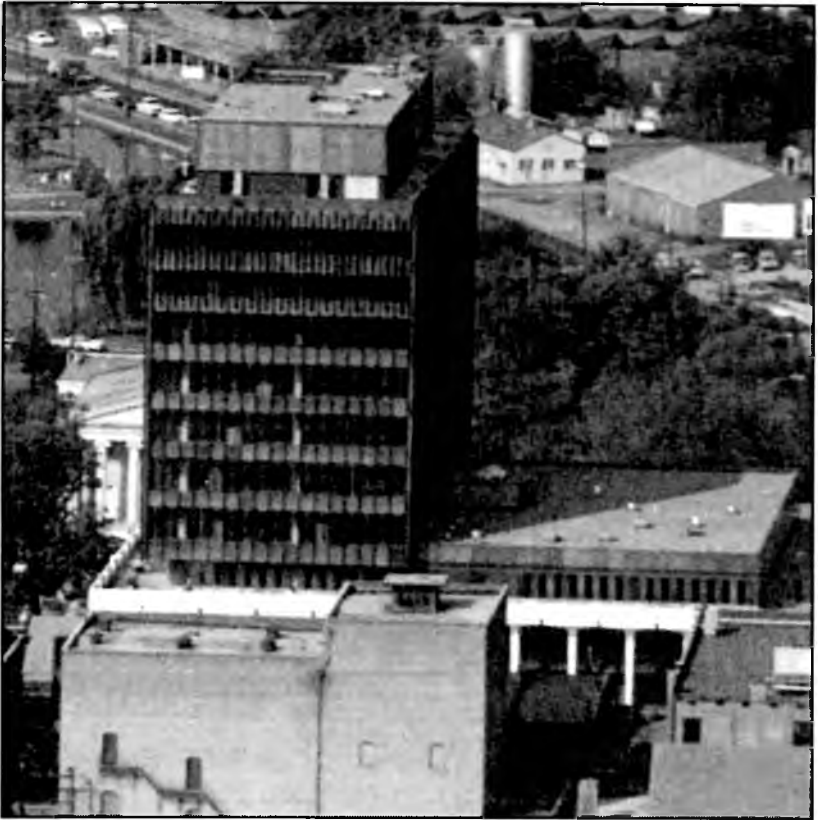
Fig. 2 View of new Huntsville-Madison County Courthouse, under construction.
