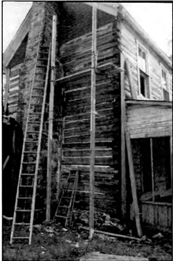
Fig. 7 Exterior of Cabaniss-Ezell House, late 1980s.
