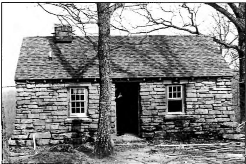
Fig.9 Cabin at Monte Sano State Park with new roof and new windows.
