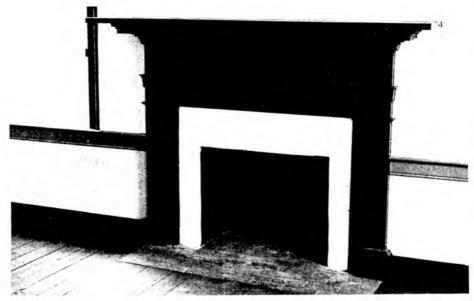
door trim. After this, the plaster was applied to the handsplit whiteoak lath or, in the case of masonry buildings, directly onto the inner surface of the solid brick walls. Therefore the plaster laps onto the edges of the wooden trim so that the trim is slightly recessed into the plaster, giving the trim a more delicate, thin appearance.
