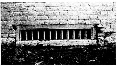
A foundation vent illustrating the diagonally placed bars and the three-quarter round mold framing the opening. Notice the Flemish bond of the surrounding brickwork.
