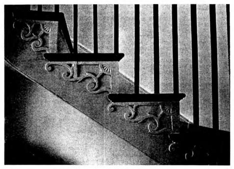
This detail of the stair scrolls shows how the pattern compresses as the stairway begins to curve.
