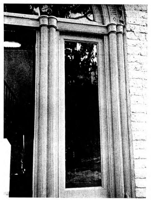
The sidelights of the front entry are flanked by extremely attenuated, reeded columns grouped in pairs. The leaded glass of the sidelights has been replaced.
