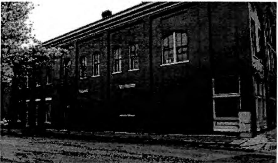
*Figure 4 — Franklin Street side of Harvie P. Jones Building showing bricked-in opening added after 1904. Courtesy Historic Huntsville Foundation files.*
