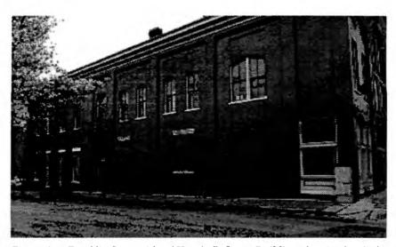
Figure 4 — Franklin Street side of Harvie P. Jones Building showing bricked-in opening added after 1904. Courtesy Historic Huntsville Foundation files.
