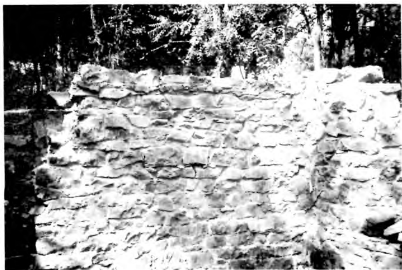
Monte Sano (Chapman) Dairy—The 19th century limestone cooling barn of the dairy sits near a springhouse and bottling barn. Before the Gladstone Place Homeowners Association stabilized the stonework in 1995, the rubble interior of the wall was exposed (top). Stonemason Robert Ervin repointed the walls with a lime-based mortar and constructed a random cement cap to stop further weather deterioration. Photos by Diane Ellis.
