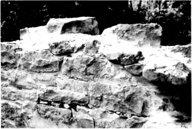
Monte Sano (Chapman) Dairy—The preserved ruins of the roughly-coursed, undressed limestone walls illustrate the vernacular use of stone. The thick stone walls also helped the dairy maintain cool temperatures for their products. Photo by Diane Ellis.
