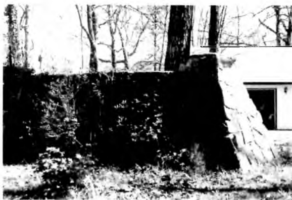
The CCCorps camp wall—Composed of stone piers with a stone wall between, the wall flanks the intersection of Highland and Monte Sano Blvd. The wall contains stone that has been surface dressed to maintain the slope of the piers but otherwise left in irregular shapes. Photo by H. Cross.
