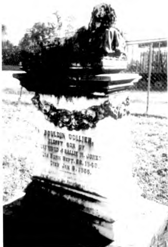
Headstone of Bouldin Collier—Signed by the A.A. Baker marble yard, this example of carved white limestone illustrates the ability of the material to withstand weathering and pollution.
