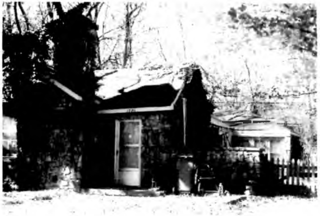
1726 Monte Sano Blvd.—The Judd home displays rubblework with thick, irregular mortar as well as rough stone window sills and lintels. Also note the flagstone path from the front door. The tile roof no longer exists and evidence of modern plumbing can be seen to the right of the door. Photo by H. Cross.
