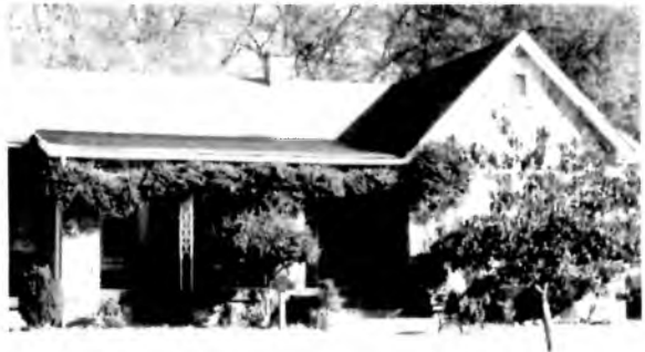
2335 Brandon—A later stone bungalow which incorporates broken range and random range ashlar as well as brick around wall openings and tile on the porch and stairs. Photo by H. Cross.
