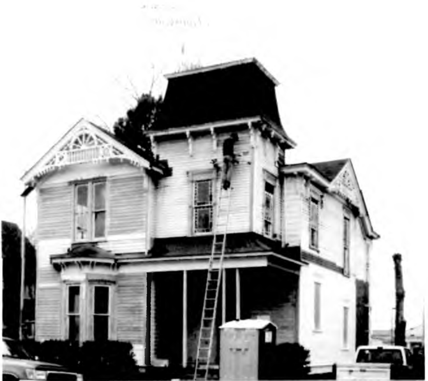
Figure 3: East front, Goldsmith-Donovan House, during restoration, December 1997. Joe Watson is atop the ladder:
