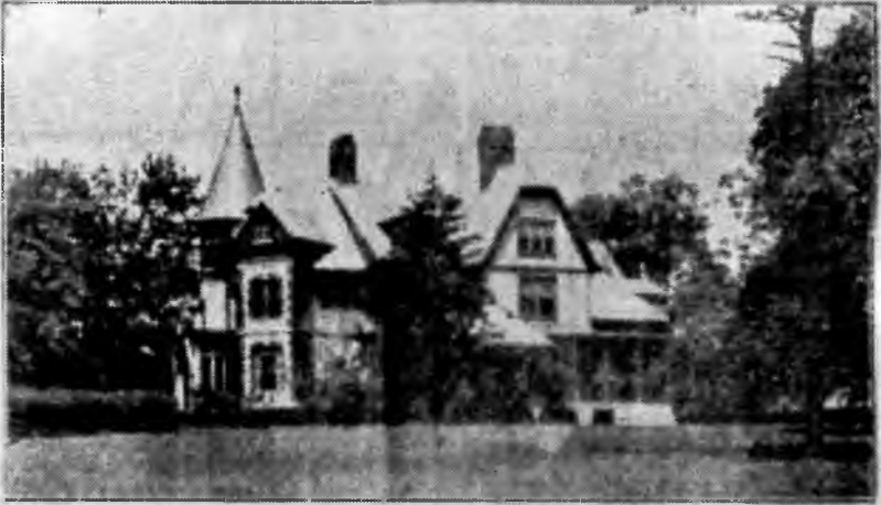
VIEW OF KILDARE HOTEL OVERLOOKING SPACIOUS GROUNDS
