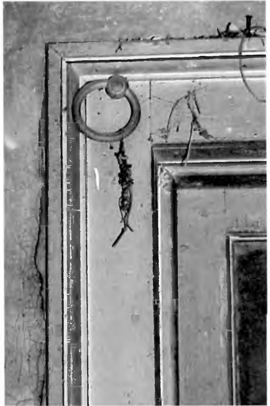
Typical Federal window and door casing. This profile is found in all rooms except the upstairs center room and the smokehouse.
