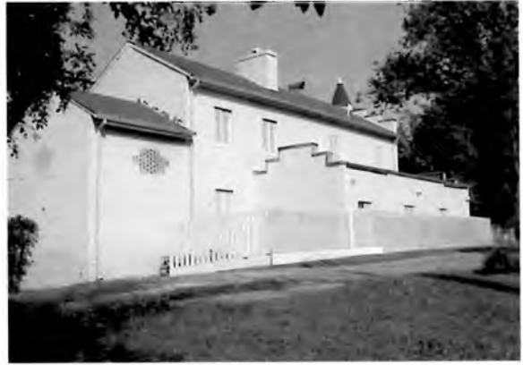
Southwest view showing smokehouse at left. One-story addition with parapet was added about 1950
