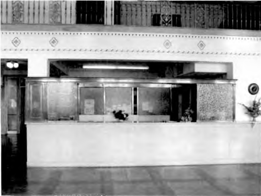
Front desk west elevation, 2004. Courtesy Fuqua Osborn Architects
