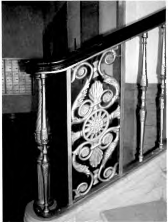
Mezzanine balustrade with lyre + sunburst + inverted lyre pattern, 2004. Hotel mailboxes in background. Courtesy Fuqua Osborn Architects. Missing in this photo is the brass ball that topped the newel. Every time someone discovered that the ball was removable, it would go missing for awhile. See the wedding reception photograph in this issue (page 44) to view both balustrades’ newel toppers in their proper places.
