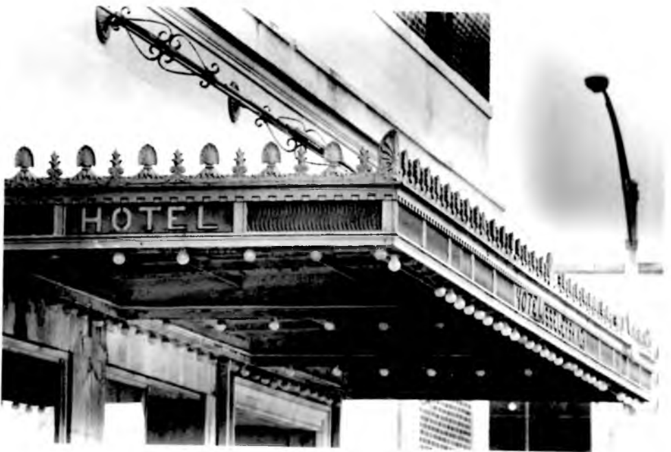
Old Clinton Street hotel marquee. Courtesy Fuqua Osborn Architects
