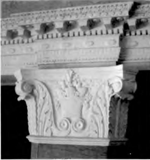
Mezzanine column capital detail, 2004. Courtesy Fuqua Osborn Architects
