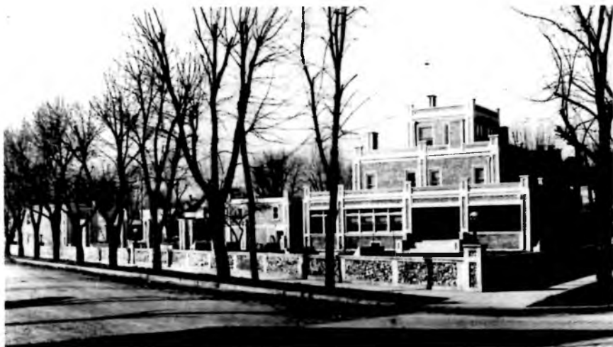
The Pierce home and outbuildings as seen when looking westward from the intersection of Holmes Avenue and Andrew Jackson Way. Courtesy Huntsville Madison County Public Library
