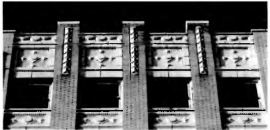
The Times Building concludes with a wide, recessed band of terra cotta, repeating the geometric pattern of the tower spandrels in an expanded design. The brickwork of the piers subtly changes at this level to accentuate a string of three-dimensional terra cotta chevrons. At the extreme top a final row of swags repeats the motif of the base spandrels. Photograph by Scott McLain
