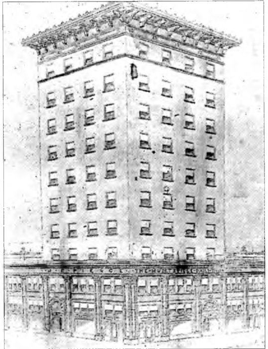
This proposal for the Times Building was published in 1925. The basic scheme is similar to the constructed building, but the built design was greatly refined using terra cotta ornament to emphasize continuous piers; the dated, overhanging cornice was eliminated; and two additional floors increased the height. Huntsville Daily Times, 28 June 1925
