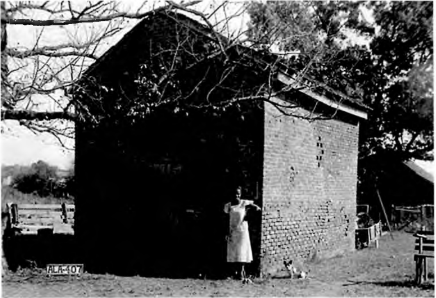
The importance of the smokehouse can be inferred by its proximity to the rear of the main house. This brick example from New Market illustrates a common local design with a vertical-plank door, diamond-patterned vents on each wall, and front gable roof. Photograph by Alex Bush for HABS, 1935
