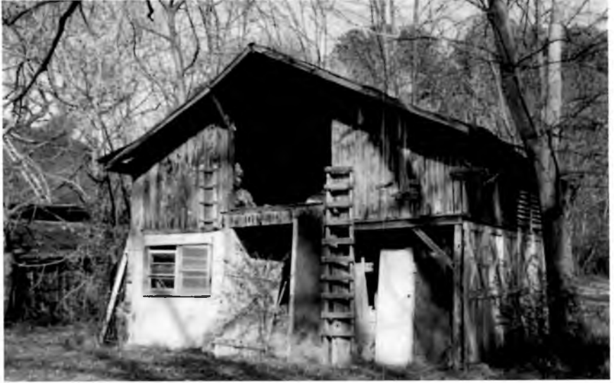
Nearby carriage house/barn showing alterations for changing uses over the years. Photograph by Linda Allen, 2004.
