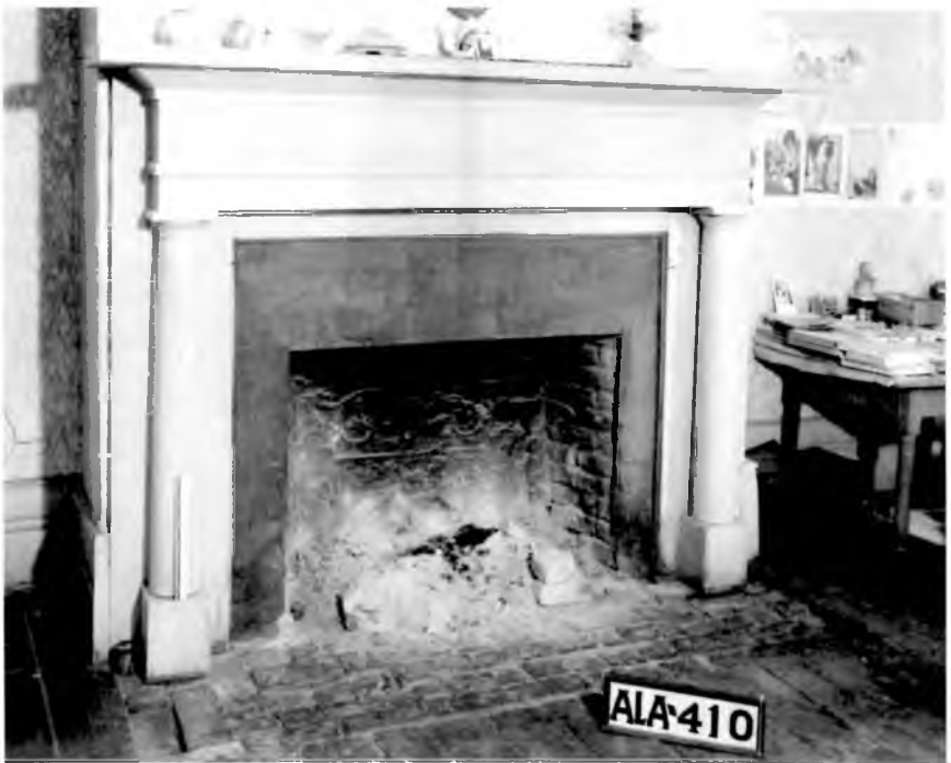
This fireplace protruded into the room and was more ornate, having an engaged column on either side. Faintly visible on the back wall of the firebox are bits of the design left by a cast iron fireback that was installed to help reflect heat into the room and protect the masonry of the chimney base. Photograph by Alex Bush for HABS, 1935
