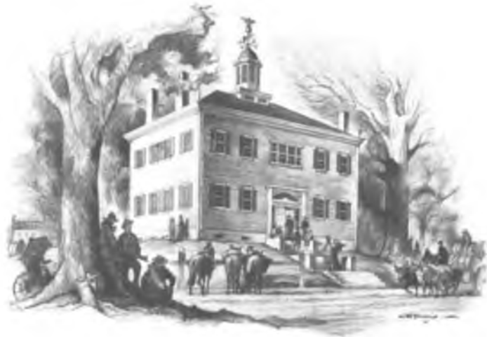
MADISON COUNTY'S FIRST COURTHOUSE
