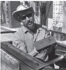
Ben Hoksbergen lifting a brick from the old sidewalk.
