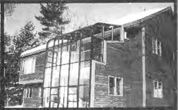
PASSIVE SOLAR GREENHOUSE: Add free solar heat and substantially reduce energy costs.
