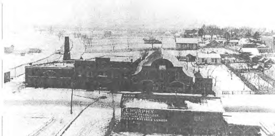
A view of the Big Spring around the turn of the century. The canal is on the left and the buildings in the background stood where Huntsville Utilities are now located.
