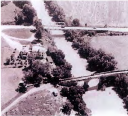
New Bridge over the Elk River
