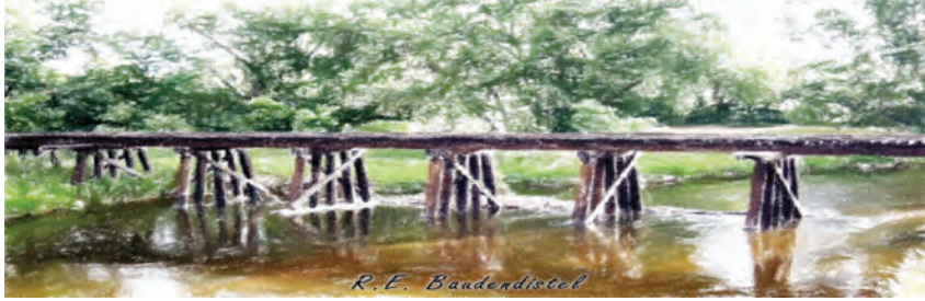
Arsenal Rail Spur Timer pile trestle spanning Huntsville Spring Branch (a.k.a) Pinhook Creek
